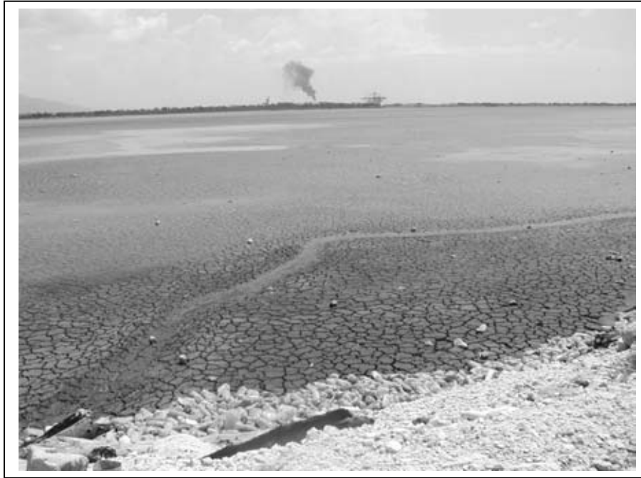
Plate 11: Area filled in with dredge spoil
