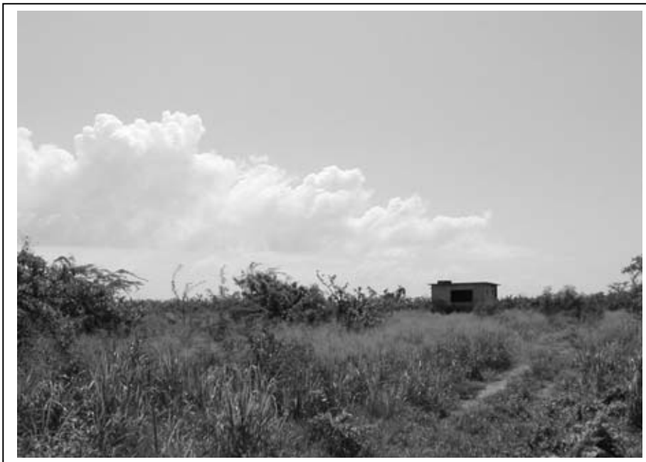
Plate 8: Old building on the property
