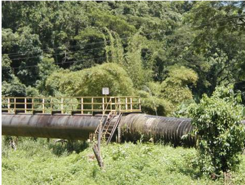
Figure 30 - Location #292 Steel section of the penstock crossing the river on a bridge
