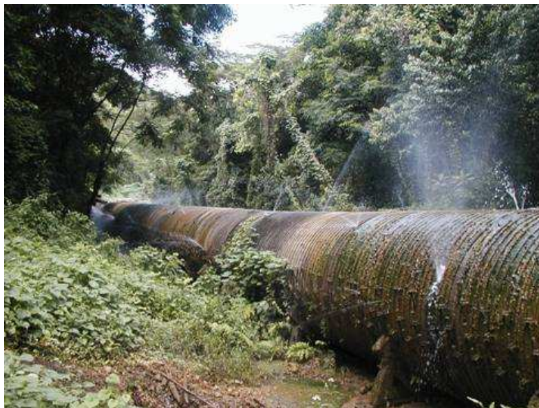
Figure 37- Location # 294 View of wood stave penstock looking upstream
