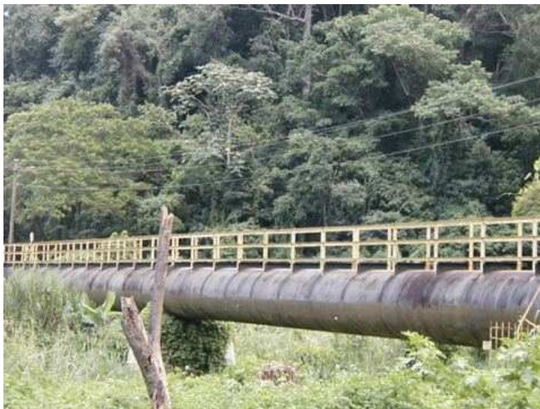
Figure 31 - Location #292 Steel section of the penstock crossing the river on a bridge
