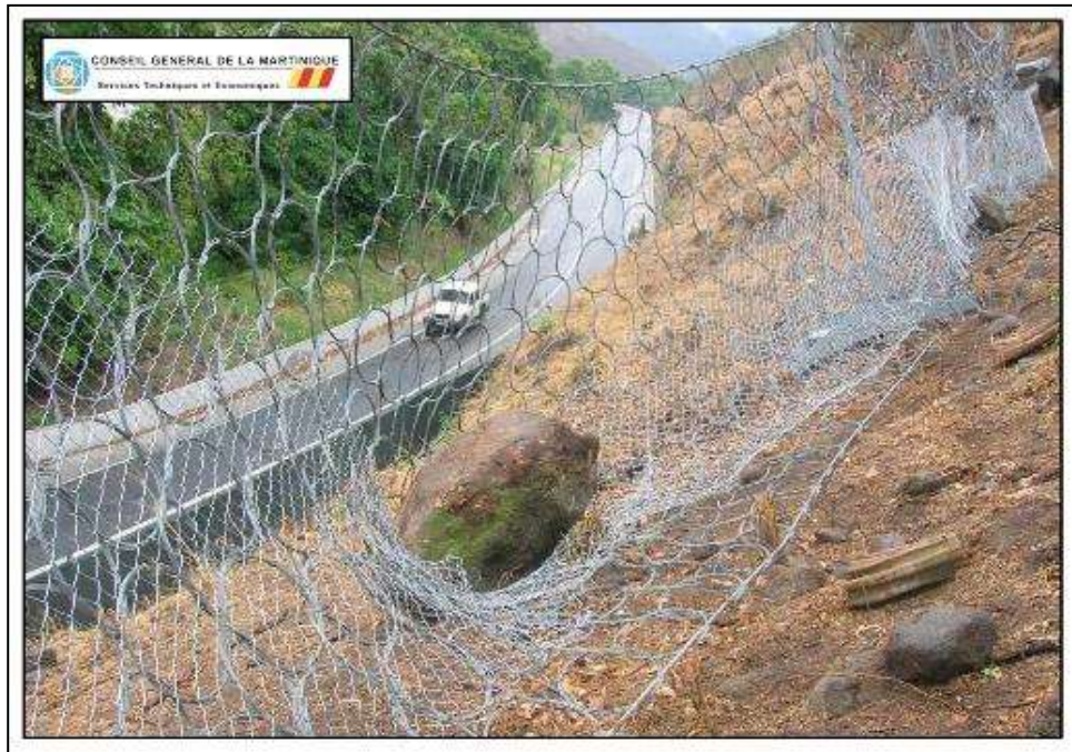
Figure 8.2.2: Example of Block Wall Net Screens for trapping boulders which are mobilized from the upper slope (Courtesy of the General Council of Martinique)
