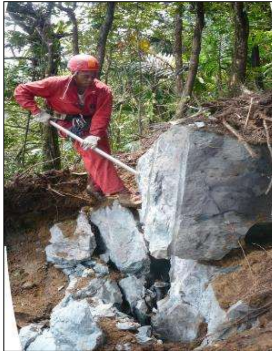
Figure 8.2.1: Manual Elimination using a miner's bar to break and remove smaller pieces of rock down the slope (Courtesy of the General Council of Martinique)
