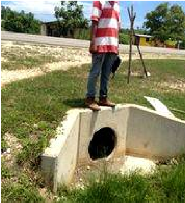
View of existing 600 mm drainage culvert which takes storm water across the main road to the coast. Note highway in background
