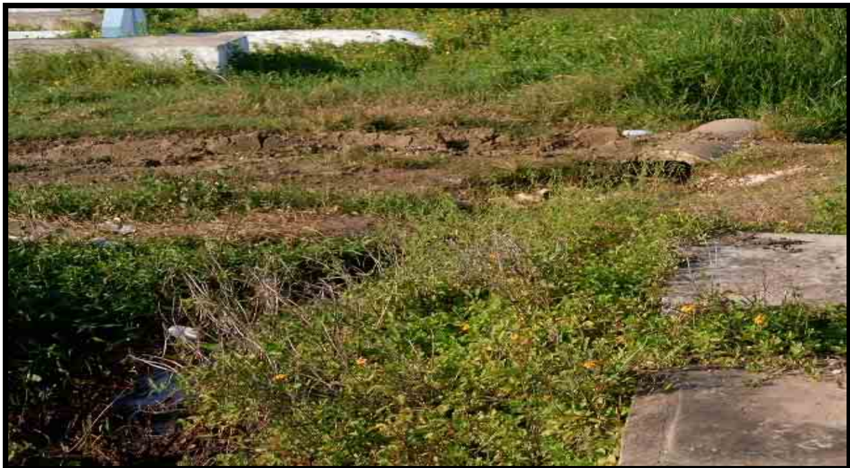
Plate 2 : Showing culvert along southward drainage channel in the Tate Cemetery
