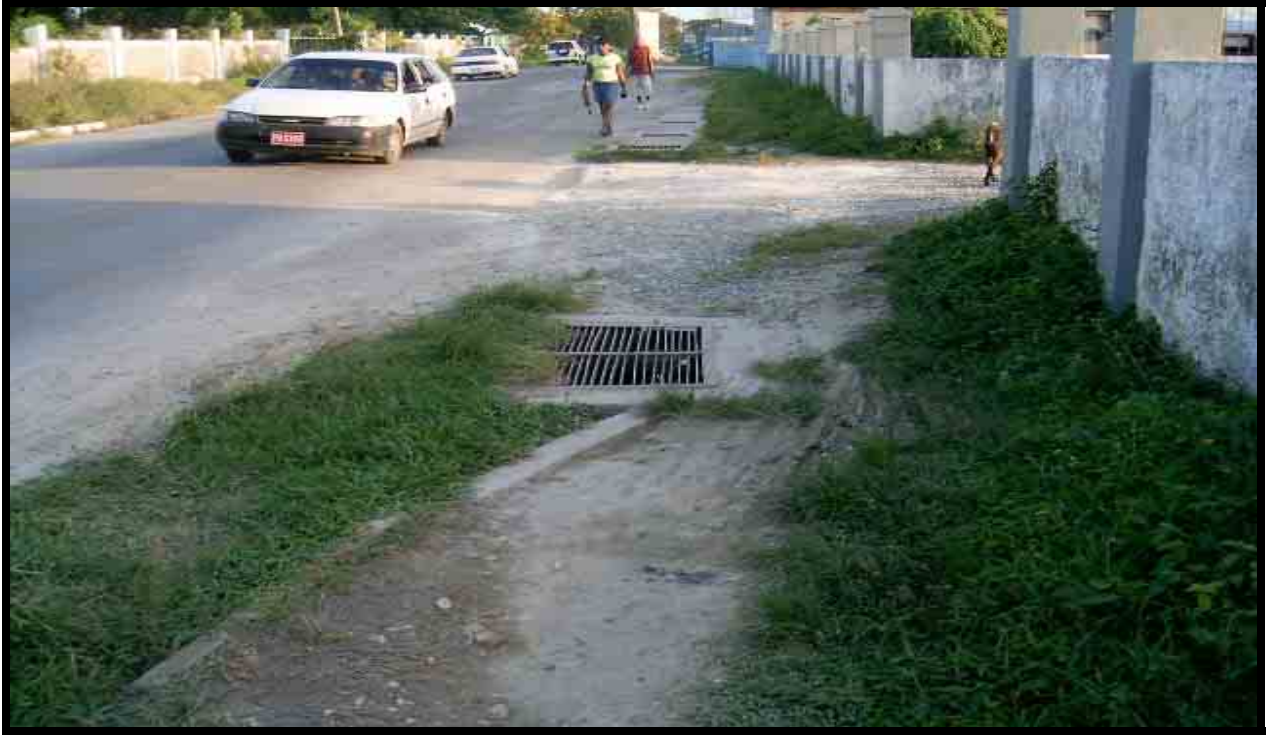
Plate 4: The system of manholes into which water runoff from the Tate cemetery is deposited.
