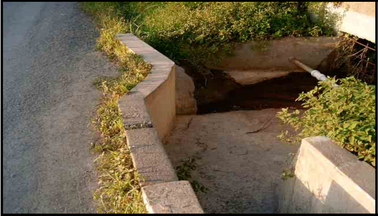
Plate 3: Culvert along Dalling Street that transports water runoff from the Tate Cemetery.
