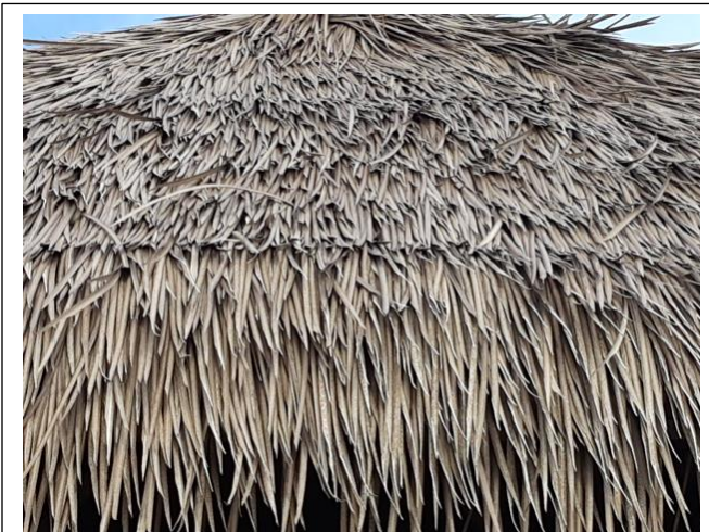
Figure: 4.21. Showing Virothatch on roof at SRC
