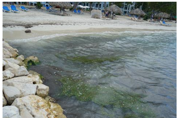
.6. Turbidity in the shallow nearshore waters. Accumulation of organic debris at the base of the groynes.
