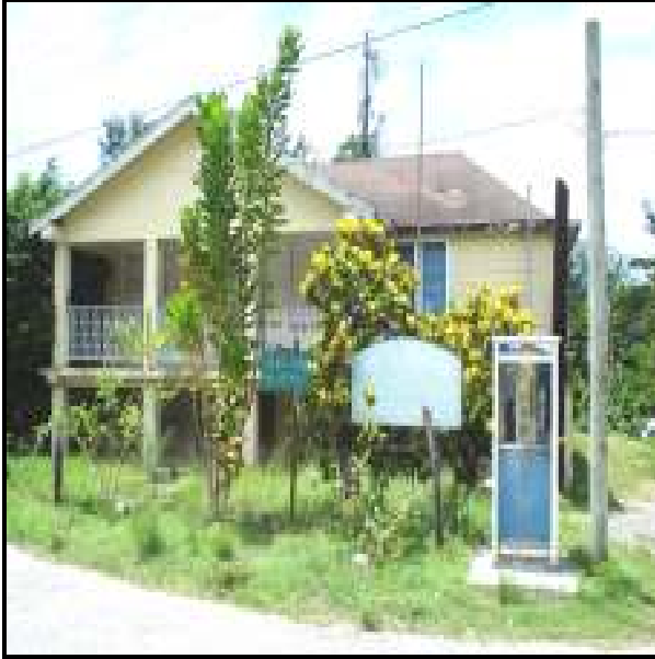
Plate 17: The old Bluefields Police Station
