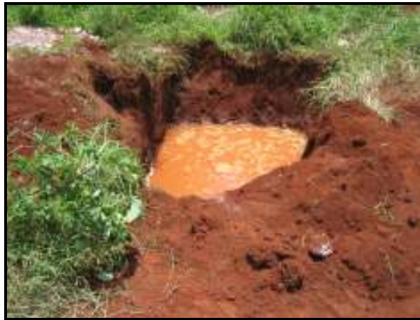
Plate 6: Test pit left to saturate before percolation test measurements are conducted. Note deep, reddish brown lateritic soil in and around the test pit
