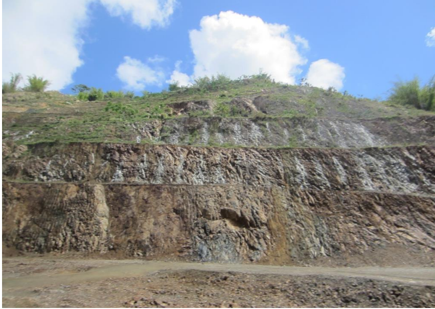
Figure 5.2: Typical Bench Slope to minimize Slope Movement, especially in deep Road Cuts
