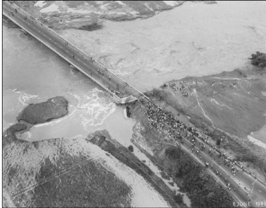
Figure 4.59: Rio Minho Highway Bridge Bypass with eastern abutment scoured out on 06 June 1986 (north to left of image)
