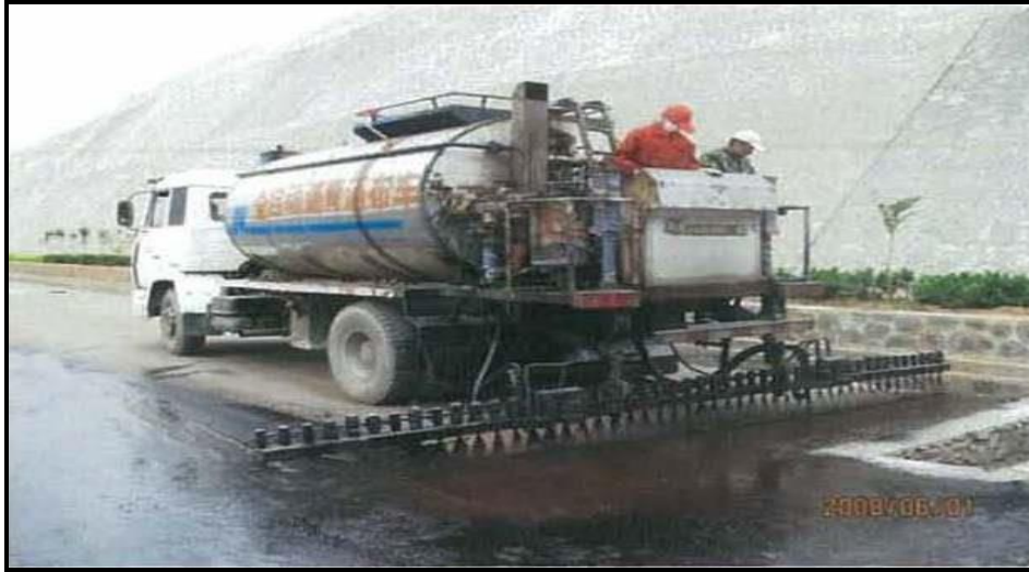
Figure 1.11: Asphalt Pavement Construction (Spraying)
