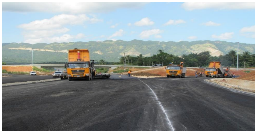
Figure 1.12: Transportation of Asphalt Concrete (Source: Mortley, 2015)
