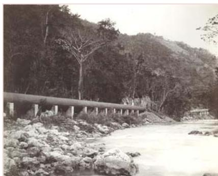
Plate 8: "The largest pipe in the world 6200 feet long 96in diameter 1700000 lbs"
