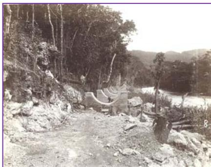
Plate 6: Concrete Pipe Saddles
