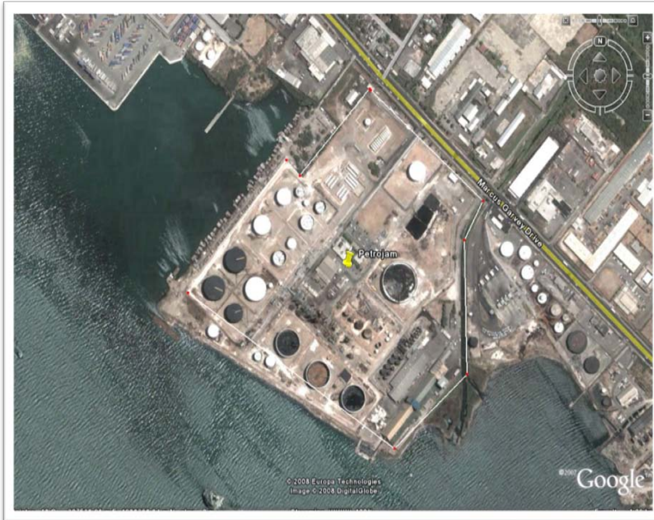
Figure 4-1 Site Location (adapted from Google Earth)
