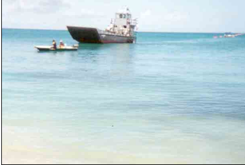
FIGURE 1-24: ILLUSTRATION OF INSTALLATION USING A LANDING CRAFT
