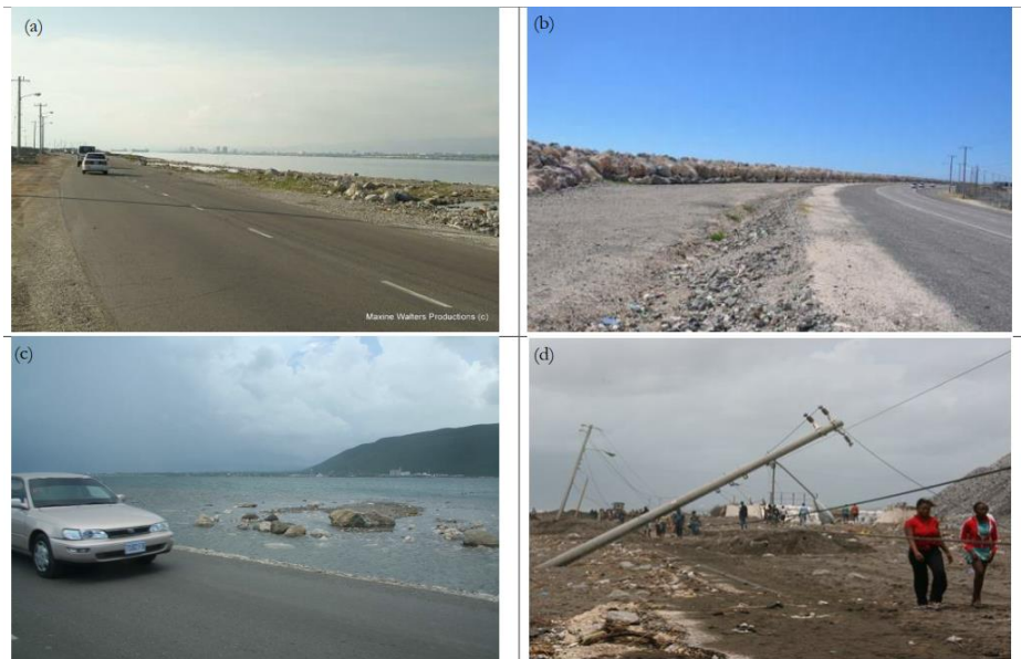
Various photos of the Palisadoes Roadway: (a) Before and (b) After the construction of the revetment; (c) right after Hurricane Ivan; and (d) after Hurricane Dean (road not shown as it is covered by washed up sand).
