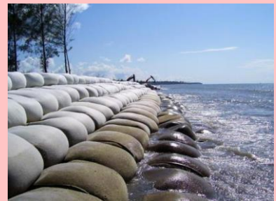
Geotextile bags used for coastal protection in the Bahamas (photo: Caribbean Geotextiles)
