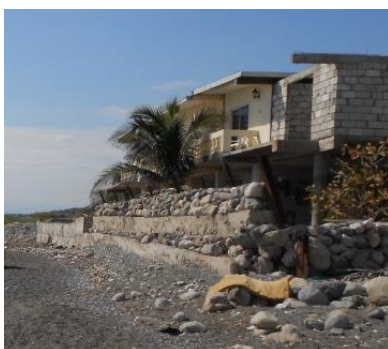
Unregulated property defence using (a) tyres at Hope Bay Beach, Portland; and (b) packed river stone at Copacabana Beach, St. Andrew
