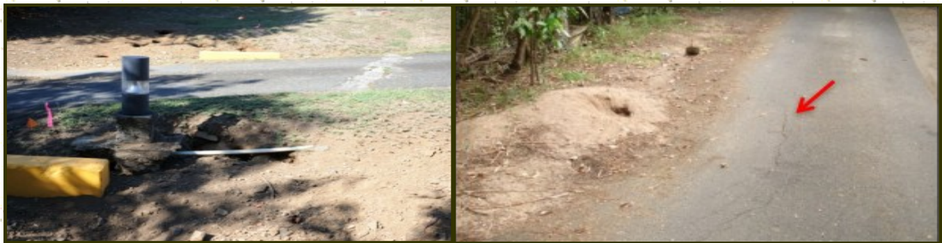
Figure 1: Damage to road infrastructure caused by Green Iguana nesting in Puerto Rico; undermining of erected structures (Left) and road collapse (right). Photographed by Carlos A. Rodriguez Gomez
