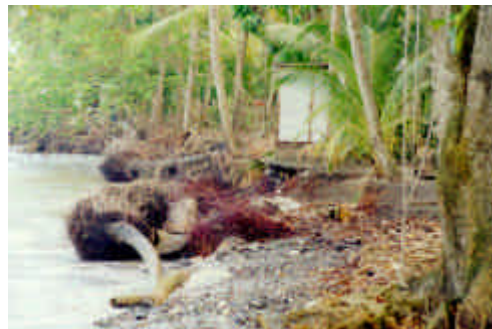
Figure 24 Beach eroded in area of concern
