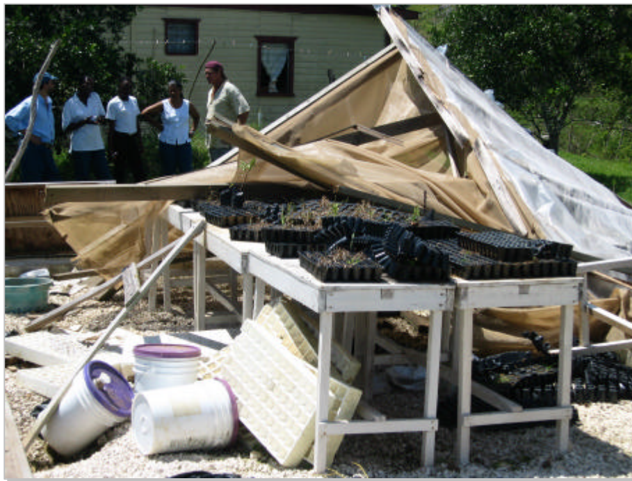
Figure 15 - Damage plant house at Cedar Grove
