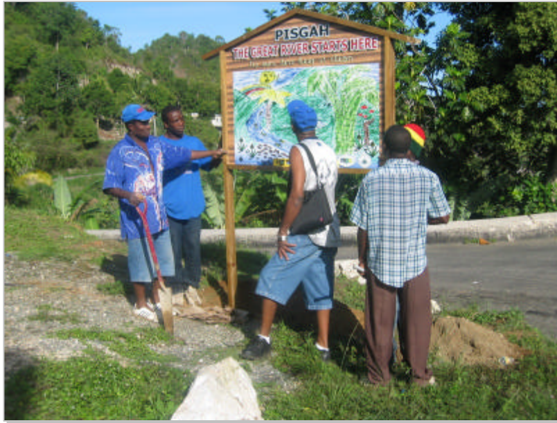
Figure 25 - Erection of the Great River watershed sign at Pisgah
