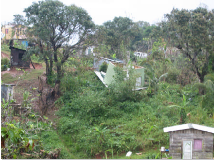
Figure 13 - Food for the poor house completely blown over in the Great River
