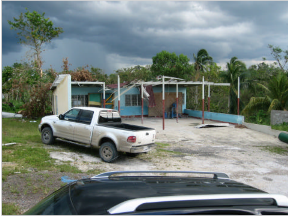
Figure 1 - Roofless meeting shed behind Cambridge Anchor Project office
