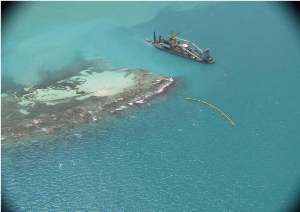
Photo #3: Silt screen on eastern side of Rackham Cay – June 16, 2002
