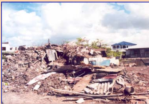
This house in Portland Cottage, Clarendon was destroyed by Hurricane Ivan
